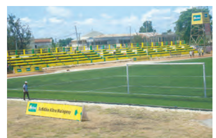
Rehabilitation of Mahajanga stadium.
